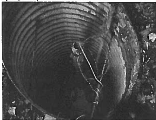
Figure 1 - Well located in a flooded well pit.
